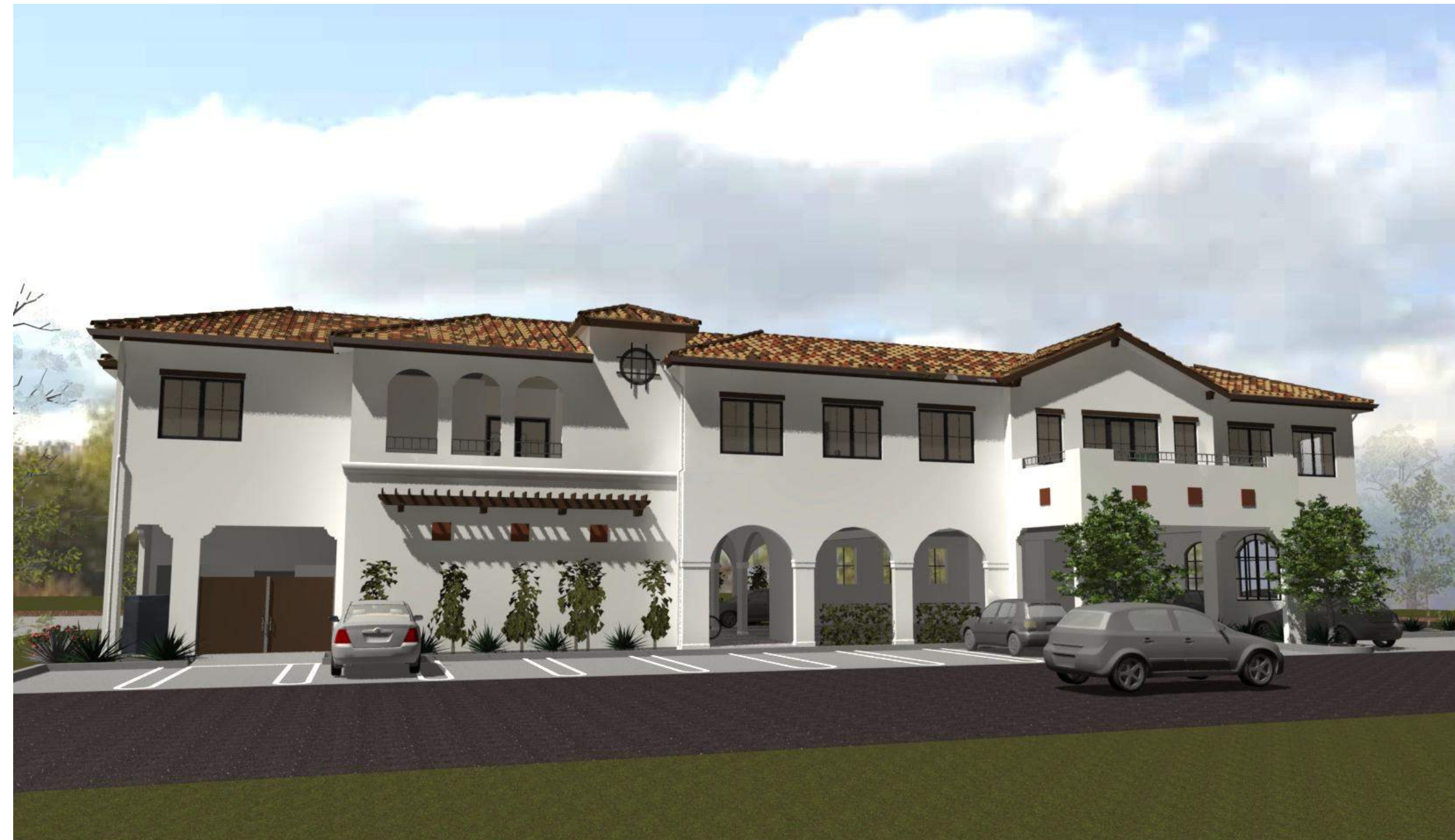
REAR VIEW - FACING PARKING LOT
